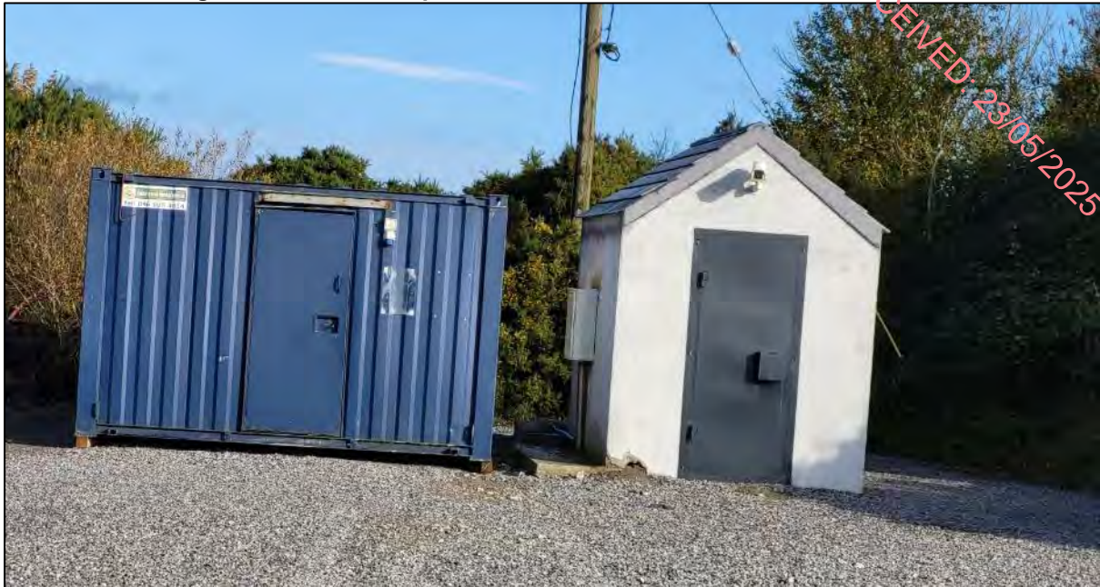
Plate 3-7: Existing Canteen and Pumphouse
