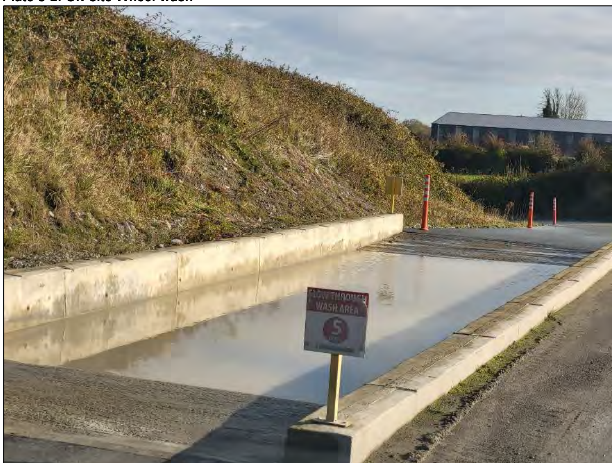
Plate 3-2: On-site Wheel wash
